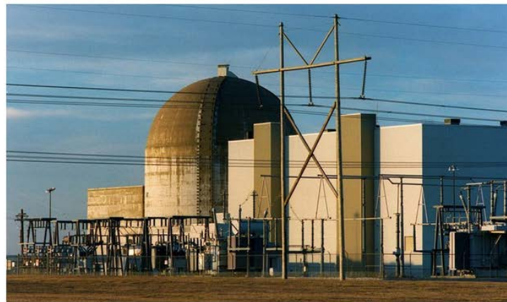
The Wolf Creek Nuclear power plant in Kansas in 2000. The corporation that runs the plant was targeted by
