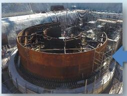
Assembly of part of the steel liner (before concrete stage)
