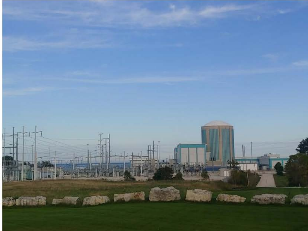
The former Kewaunee Power Station, as of Sept. 24.
