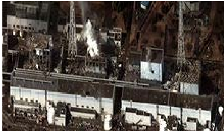
The Fukushima I Nuclear Power Plant after the 2011 Tōhoku earthquake and tsunami. Reactor 1 to 4 from right to left.
